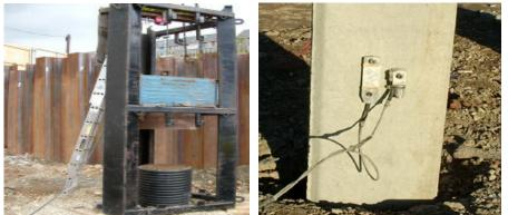
As Dependent upon the method employed, electronic gauges are attached to the pile as illustrated in side picture. The gauges measure the acceleration of the pile (and therefore (indirectly) velocity with a knowledge of the pile properties) and strain within the pile just below the head as the hammer strikes the pile. The information is then recorded in the associated site computer. A variation of the method involves deflection measurement directly by laser theodolite.
